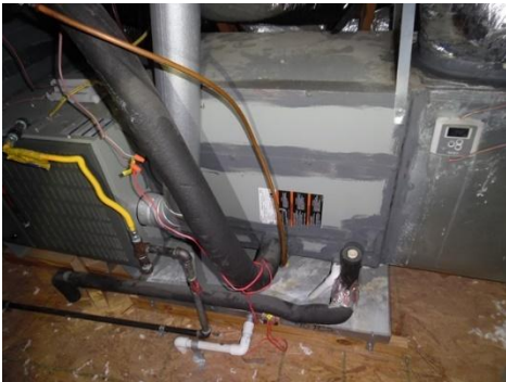
evaporator coil
