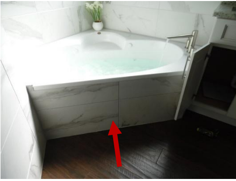
No pump and motor access
