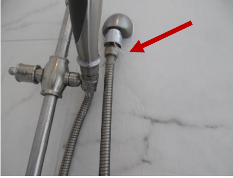
Hose connection leaks
