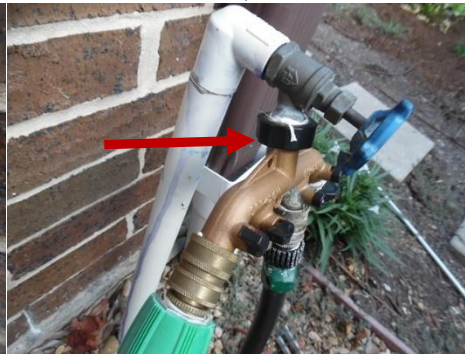
no anti siphon device
