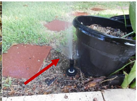
sprinkler head shooting straight up
