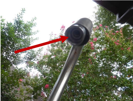
Aerator screen missing
