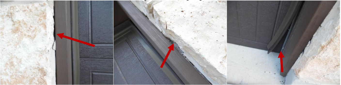
Gap is not caulked and sealed
