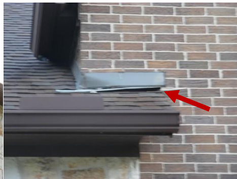
raised roofline flashing
