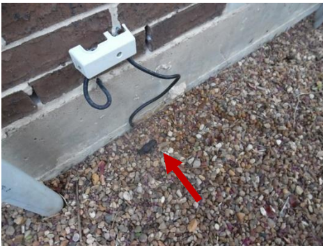
Ground rod connection below grade
