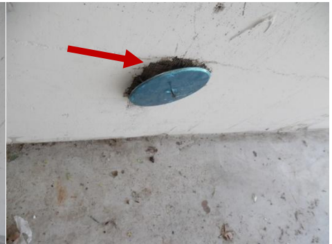
trap cap not secured to wall
