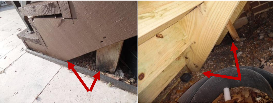
Wood to soil contact
