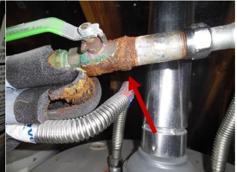
rusted and corroded water valve
