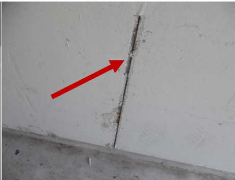
sheetrock not taped and floated
